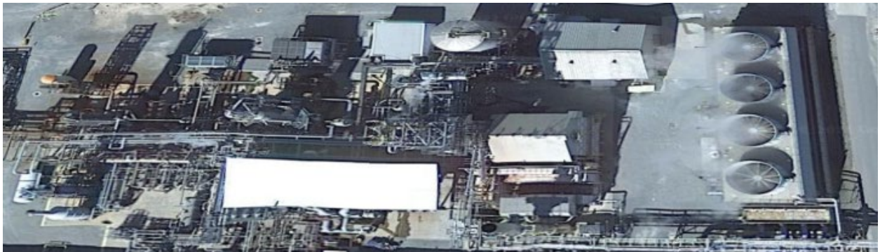
EDCC Ammonia Plant
