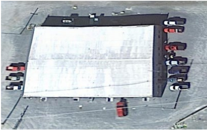
Acid / Prill Production Control room
